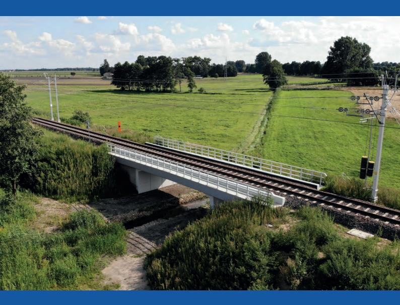
PRECAST CONCRETE FRAME BRIDGE SYSTEM
